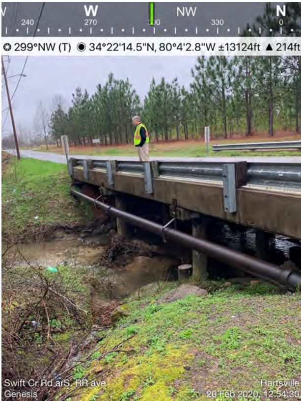
Photo 15 – Railroad Avenue bridge over Snake Branch looking at upstream side.
