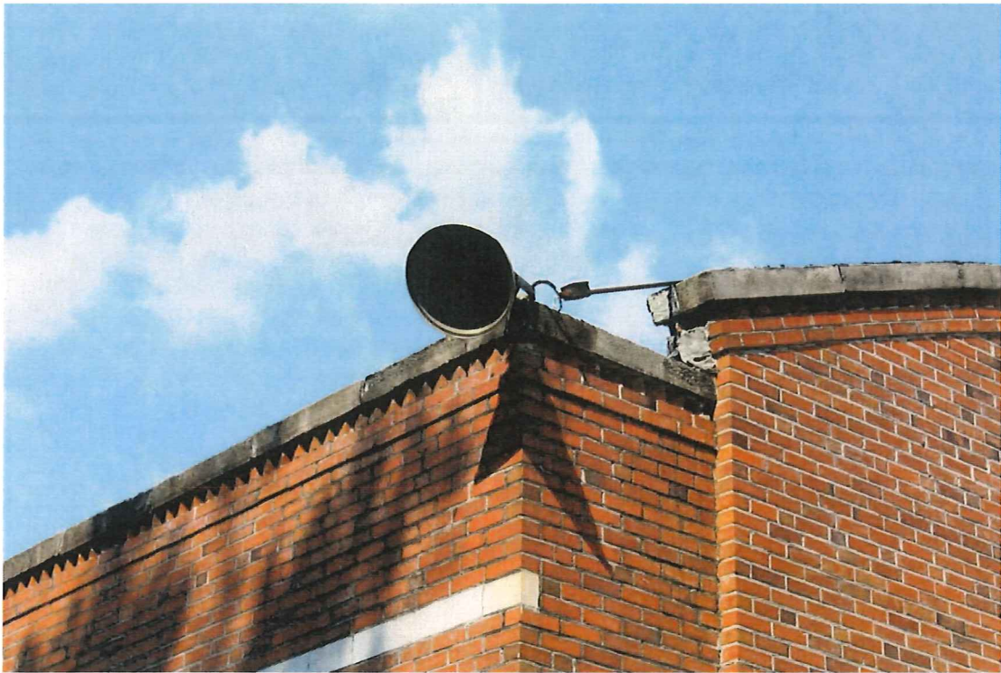
Photo 20 – Siren at southwest corner of building
