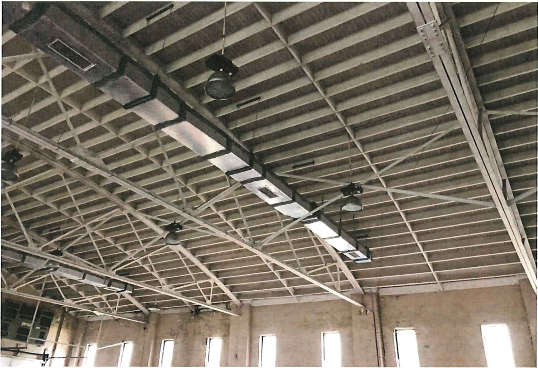
Photo 37 – Exposed trusses in drill hall
