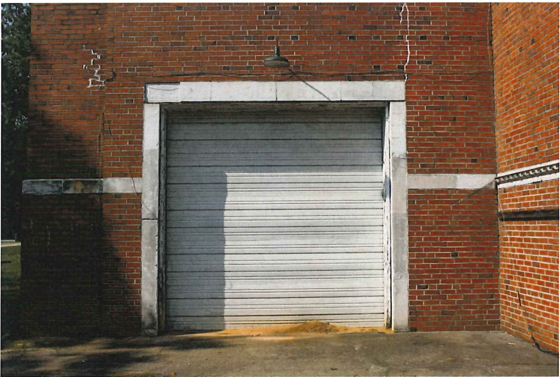
Photo 19 – Garage door at southwest corner
