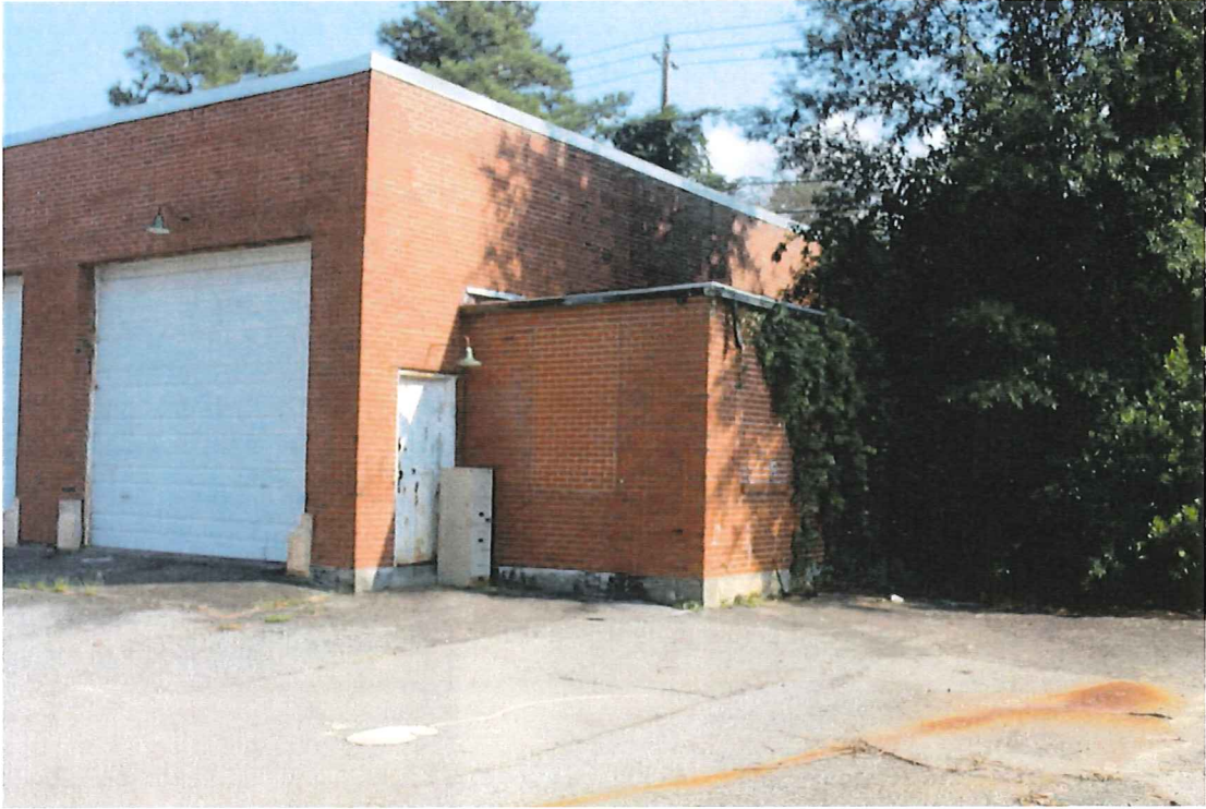
Photo 22 – Southwest corner of garage
