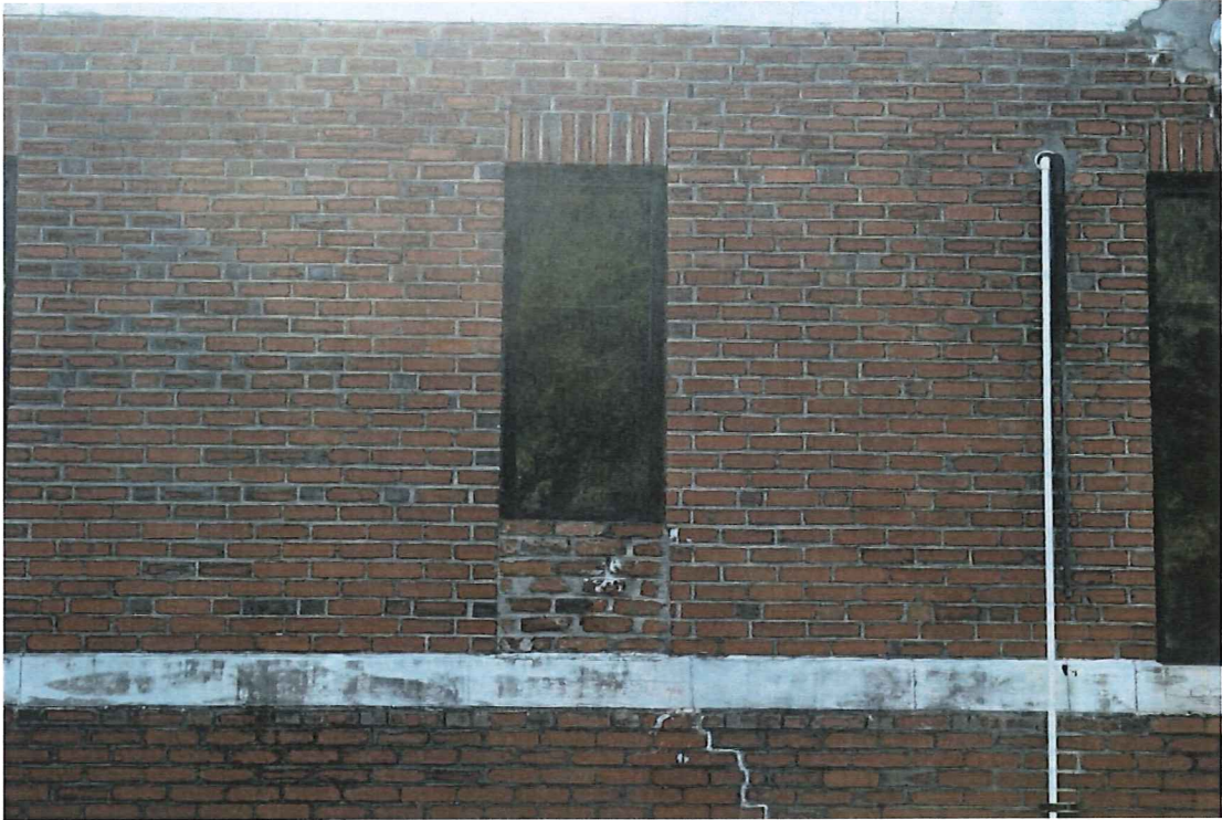
Photo 17 – Post-1994 replacement windows, drill hall
