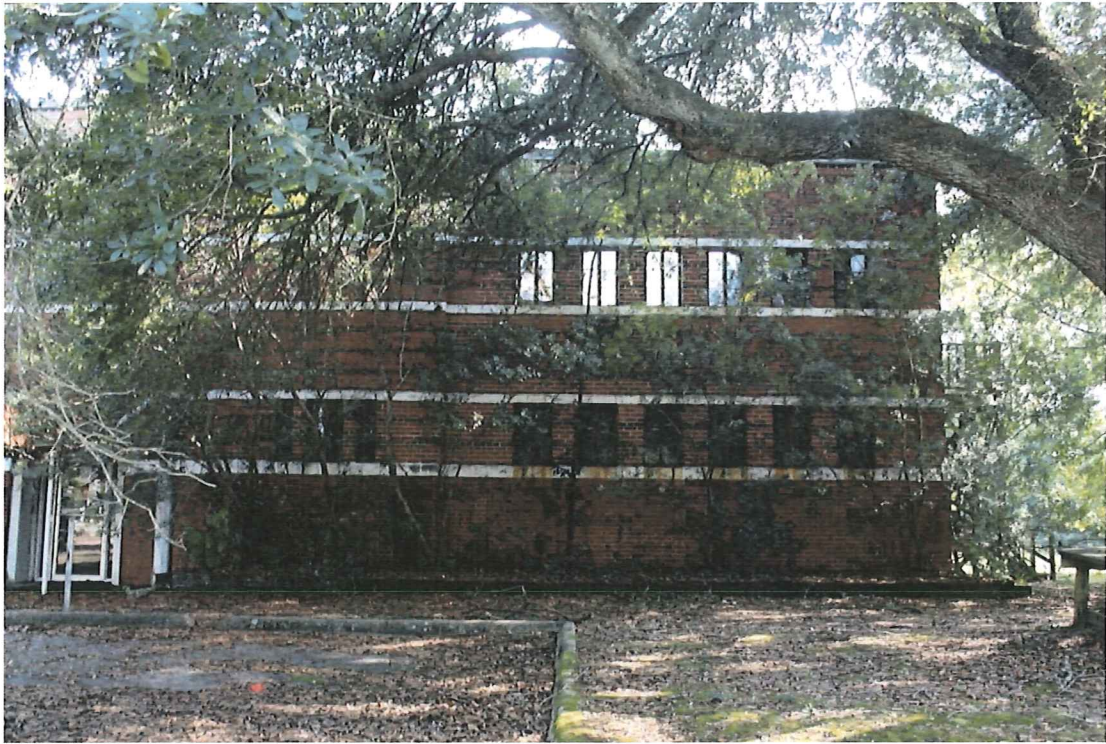
Photo 2 – West end of north façade, original windows and window pattern
