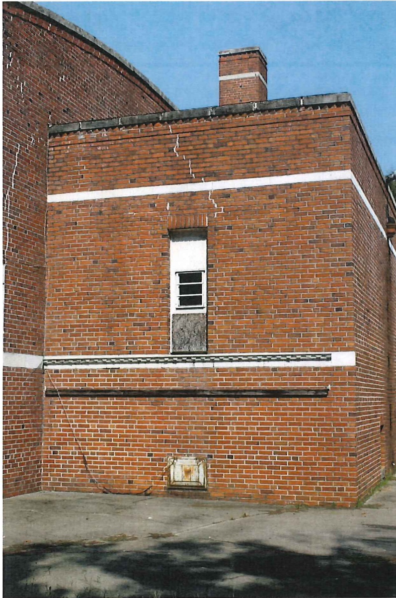
Photo 16 – Replacement window at rear stage, southwest corner
