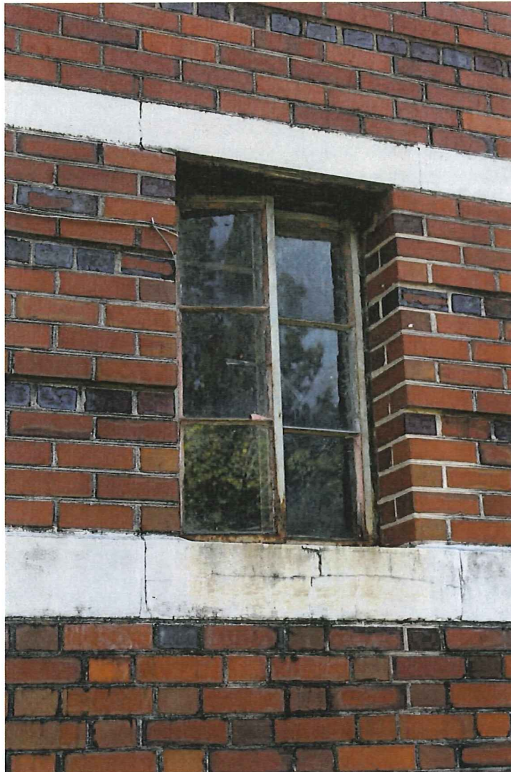
Photo 14 – Paired casement windows, west elevation
