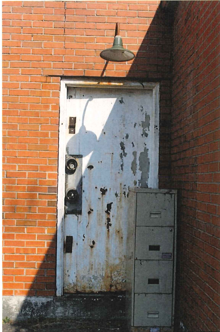
Photo 25 – Pedestrian door to garage with gooseneck light
