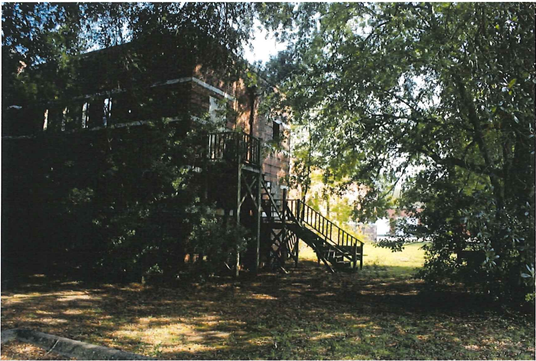
Photo 3 – West elevation with deck on administrative wing
