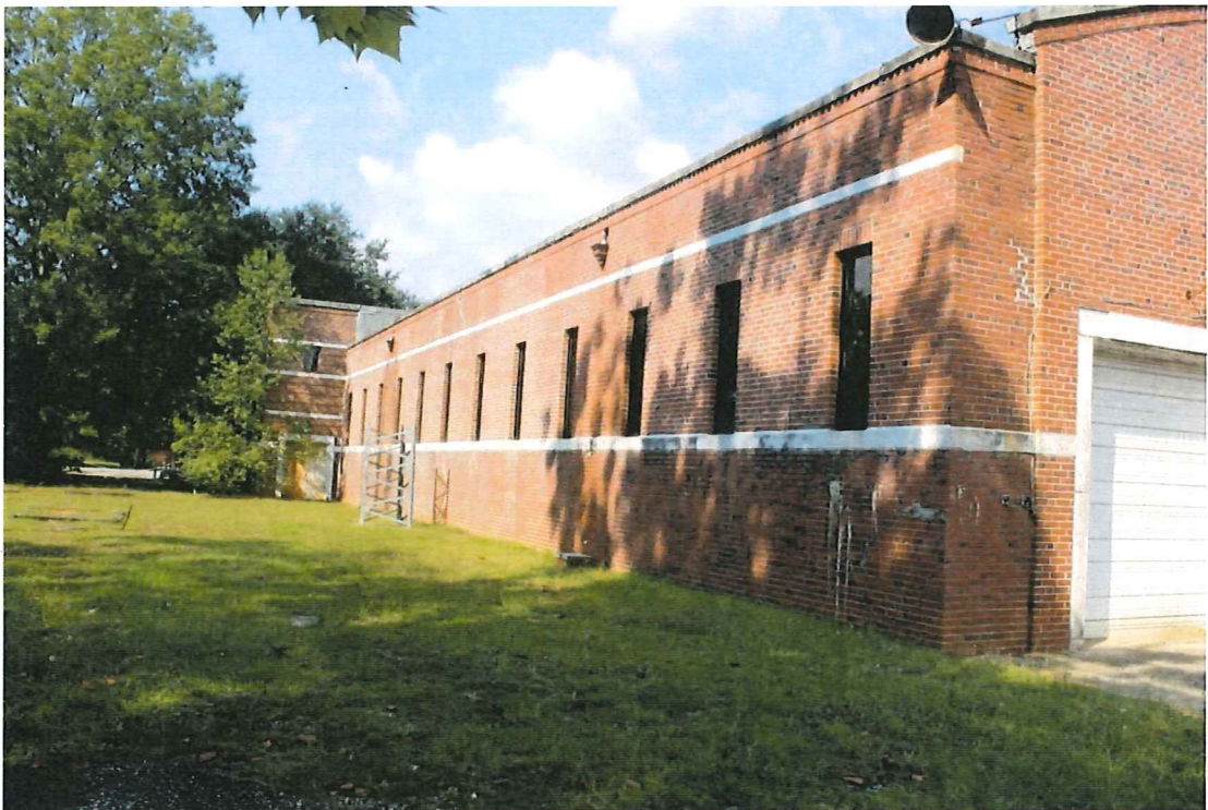
Photo 5 – West elevation looking north
