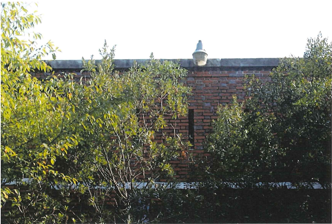
Photo 18 – Front parapet with saw-tooth corbelling and cast stone coping
