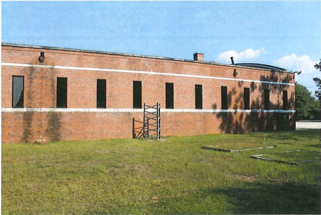
Photo 4 – West elevation of drill hall with replacement windows
