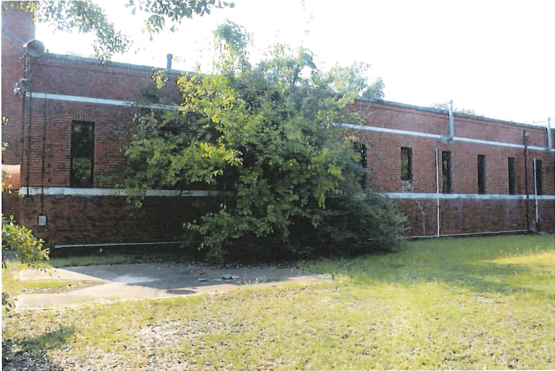
Photo 8 – South end of east elevation
