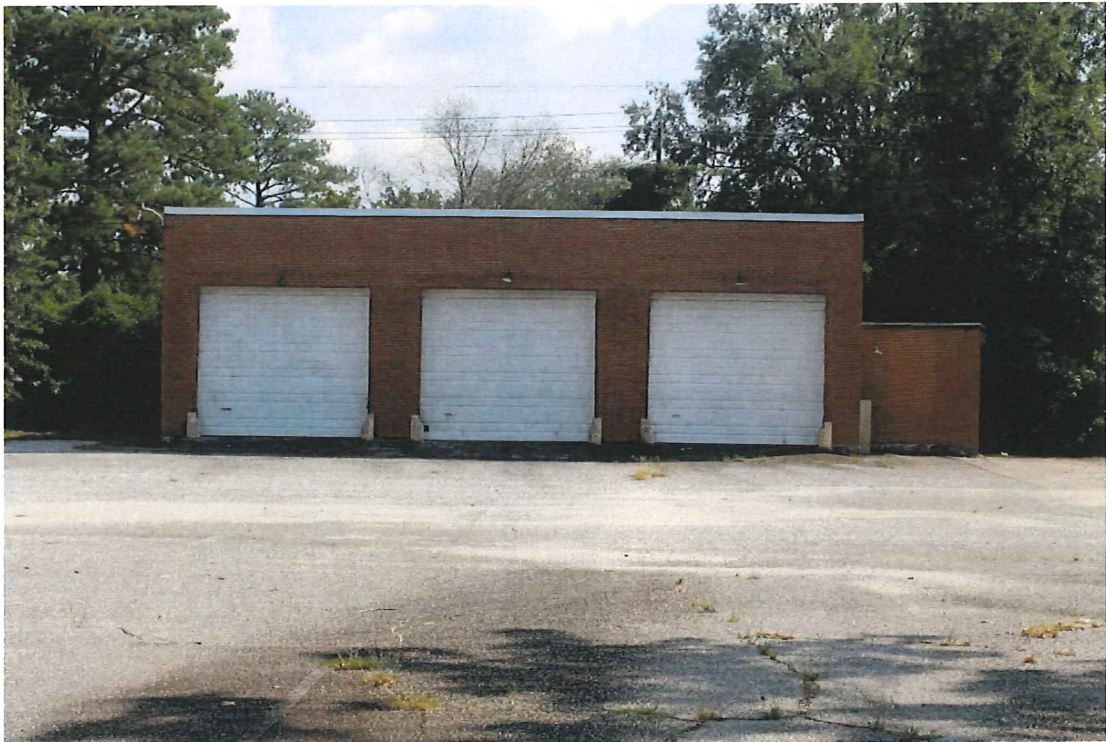
Photo 11 – Rear garage, north elevation
