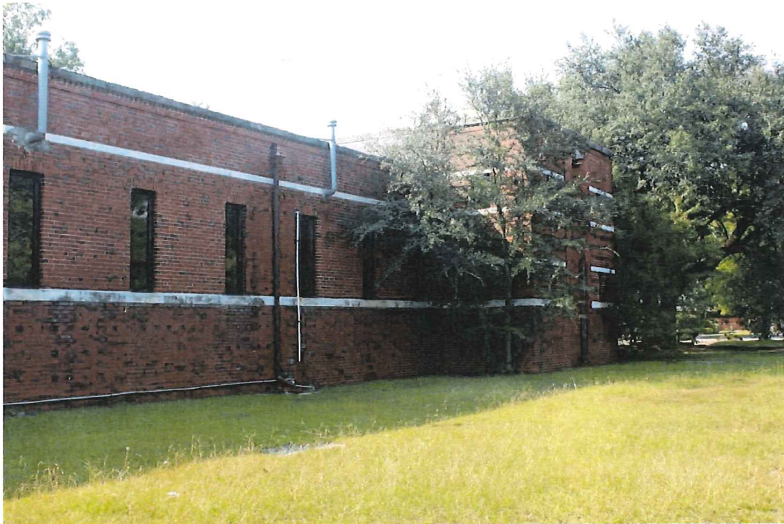
Photo 9 – North end of east elevation
