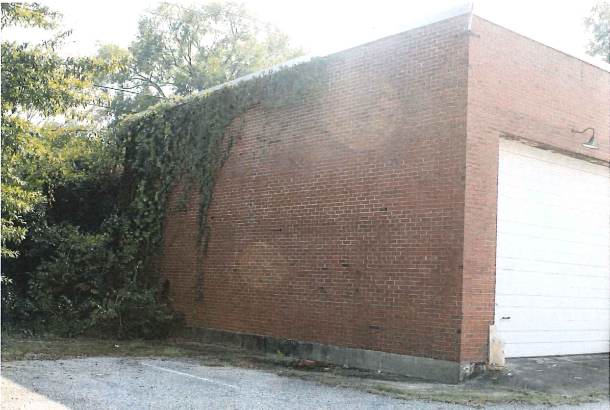
Photo 23 – East elevation of garage
