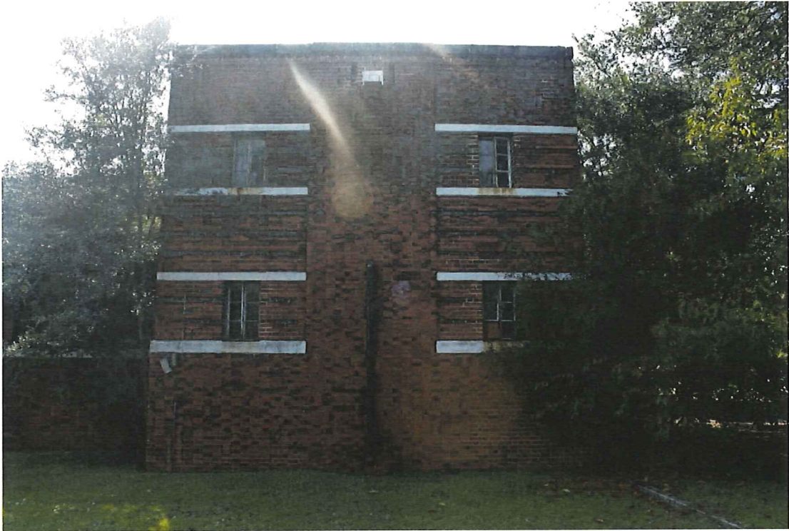
Photo 10 – East elevation of administrative wing
