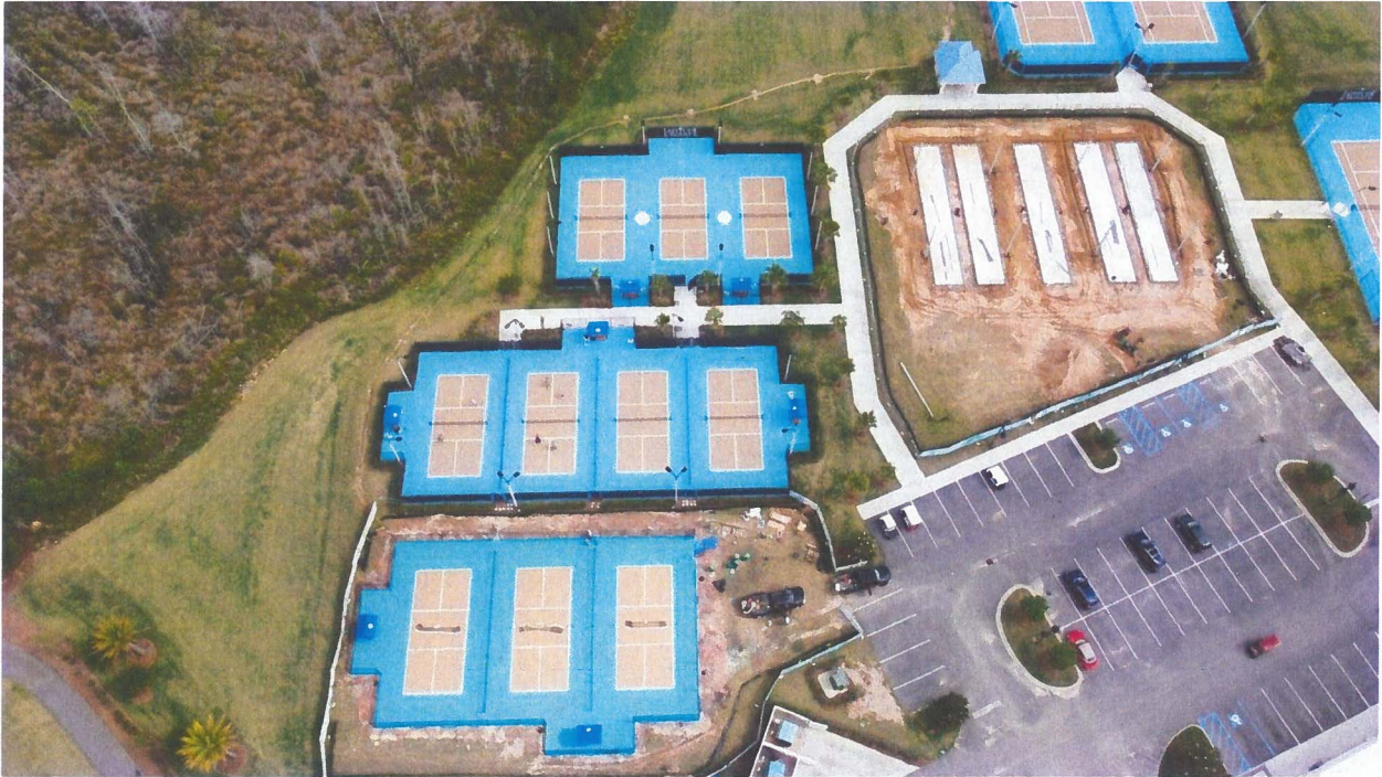
Monroe High School – Albany, GA – 2018 - JCI Contractors - Jason Norris - Constructed a Triple Tennis Courts – Our scope of work including fine grading the subgrade, installation of GAB and paving, Fencing, Surfacing and Striping and Tennis Court Accessory's.
